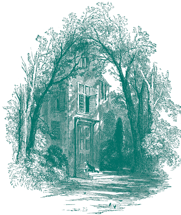
Sheltering in Place
