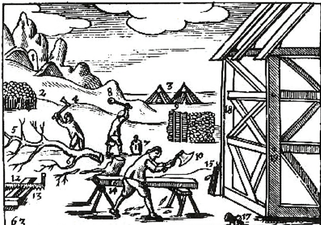
Figure 1.—1685: THE PRINCIPAL TOOLS that the carpenter needed to frame a house, as listed by JOHANN AMOS COMENIUS in his Orbis Sensualium Pictus were the felling axe (4), wedge and beetle (7 and 8), chip axe (10), saw (12), trestle (14), and pulley (15). (Charles Hoole transl., London, 1685. Courtesy of the Folger Shakespeare Library.)
